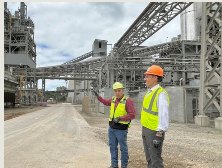
Midwest Region | Mitchell Cement Plant
