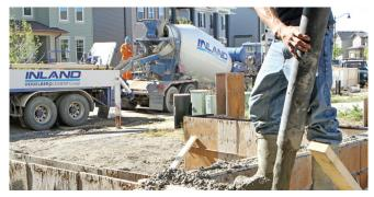
Inland Concrete offers our Redi-Slump mixes with a pre-engineered slump that arrives on site at the customer desired slump range. Unlike the traditional method of adding a high range water reducer (HRWR) or super plasticizer at the site, which is known to cause inconsistencies, Redi-Slump is engineered to produce desired slumps directly from the concrete plant.
