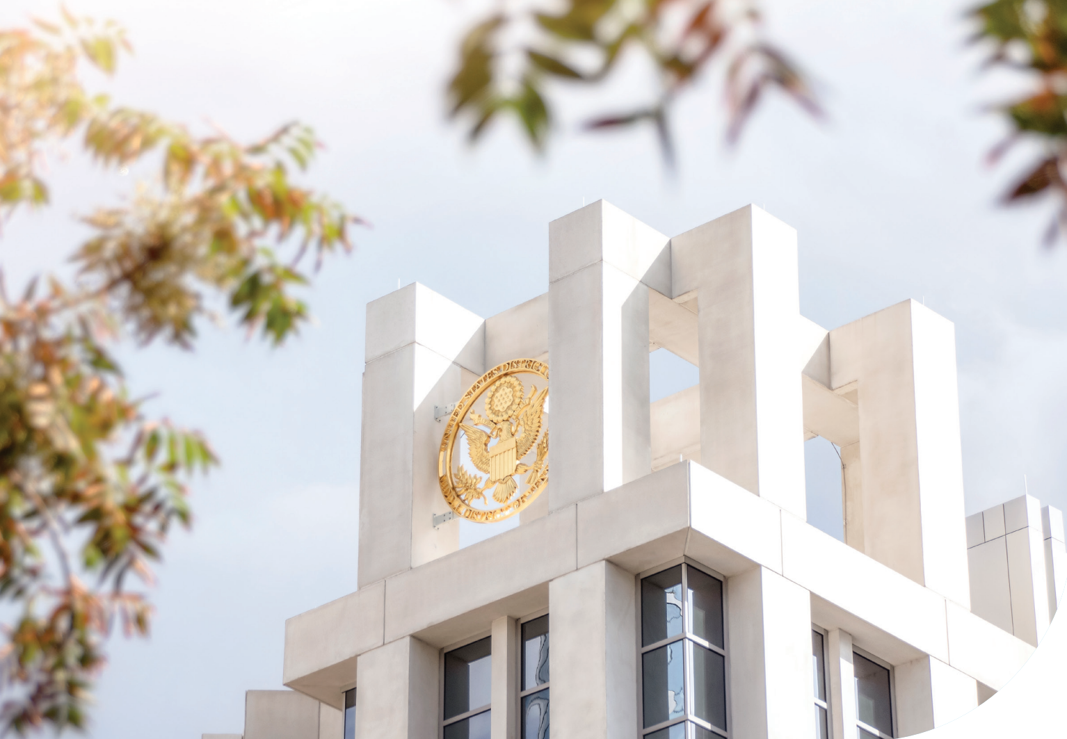
The Fred D. Thompson U.S. Courthouse in Nashville, TN, pictured above, is the largest TX Active project to-date in the world.
