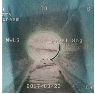
Differential settlement has caused this grouted flexible connection to separate.
