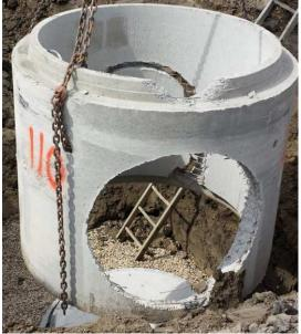
Barrels are specially designed for each project to ensure the cores don't impact the structural integrity of the manhole.
