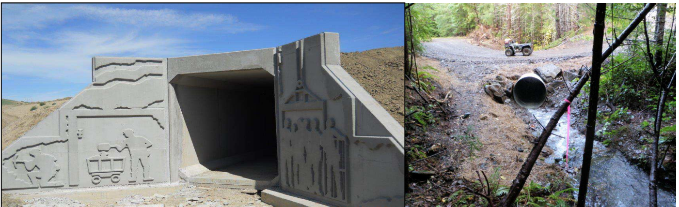
Left: In addition to offering improved hydraulic performance, precast concrete headwalls are also aesthetically pleasing. Right: A typical CSP inlet with no end treatment.
