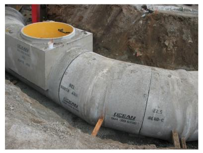
Ocean Pipe chose to line the pipe using AGRU 2mm high density polyethylene liner. The AGRU liner was chosen for two reasons: the HDPE was stiffer than other products on the market which made it easier to work with during manufacturing, and the v-shaped anchor system, a patented AGRU system known as Sure-Grip, allowed for a more uniform embedment within the concrete pipe than other anchor systems.
