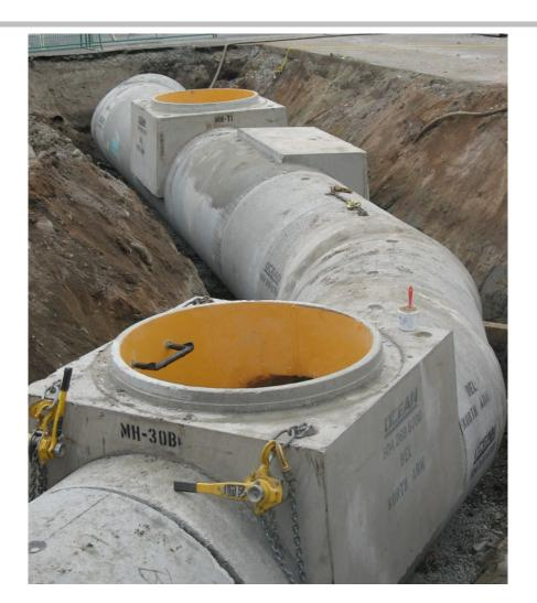
The North Arm Interceptor Project involved the relocation of an existing Metro Vancouver owned sanitary sewer line located at 1041 SW Marine Drive. The new line was to be 1350mm diameter concrete pipe with a plastic lining to negate the potential for corrosion due to hydrogen sulfide growth. Construction began in late July and was completed in September 2014.
