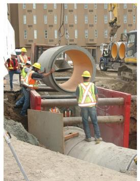
of twenty-one specialty/fittings pieces and thirteen standard lengths of straight pipe. A total of twelve single mitre bends, five manhole tees, two steel wyes off concrete pipe which were used to bypass the existing line into the new one, and four custom-length pieces were all created for this sanitary line.
